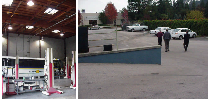
Inadequate vertical clearance for lifts, ventilation, etc., and entry slope.
