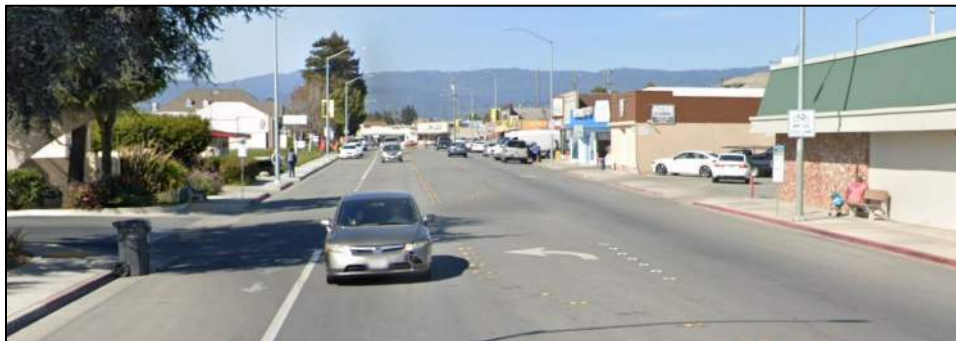
Bus Stop Adjacent to a Side-street Stop-Controlled Intersection without a Crosswalk at 1003 Freedom Boulevard, Watsonville, CA
